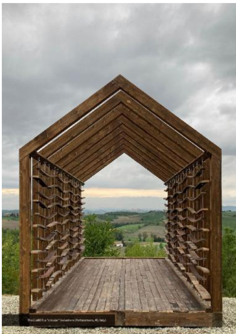
Figure 3. Picture of the CiaBOT belvedere (Source: https://riunet.upv.es/entities/publication/2bff1fed-68c7-43e4-acd1-da33351b32b3 )
