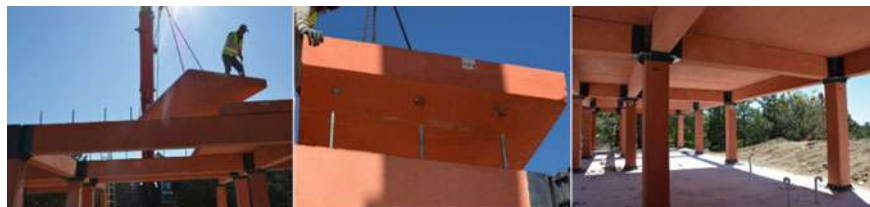
Fig. 14.9 Installation of slabs
