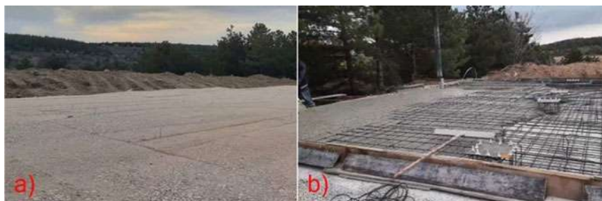
Fig. 14.5 Construction of the mat foundation, a laying of gravel; b building of the foundation
