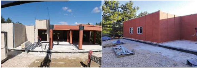
Fig. 14.10 Installation of non-structural elements
