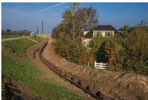
Fig. 3.7 Dyke reinforcement with sheet piles in Wolferen-Sprok [20]
